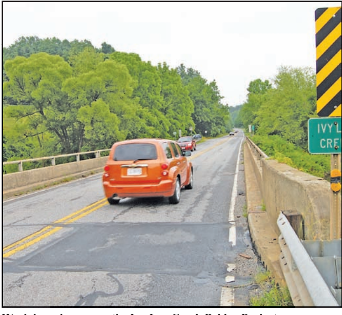
Work is underway on the Ivy Log Creek Bridge Project.
