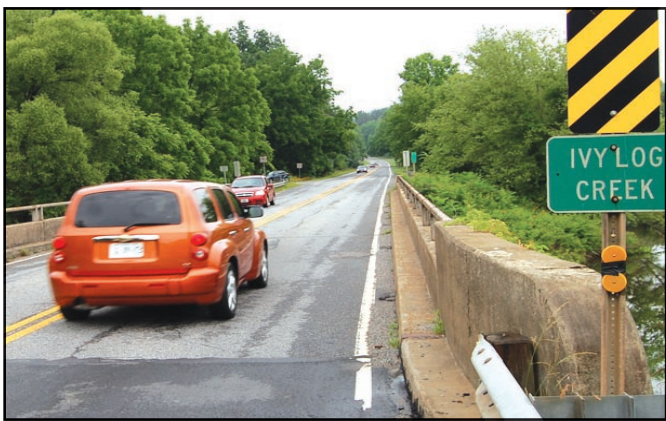
Construction will begin later this summer on a new bridge over Ivy Log Creek according to GDOT. Photo/Lowell Nicholson
